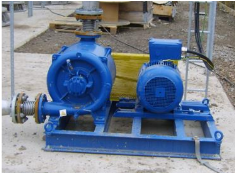
Photo 2: Standby Fan inspected every four years
