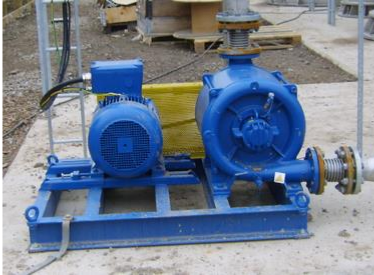
Photo 2: Standby Fan inspected every four years
